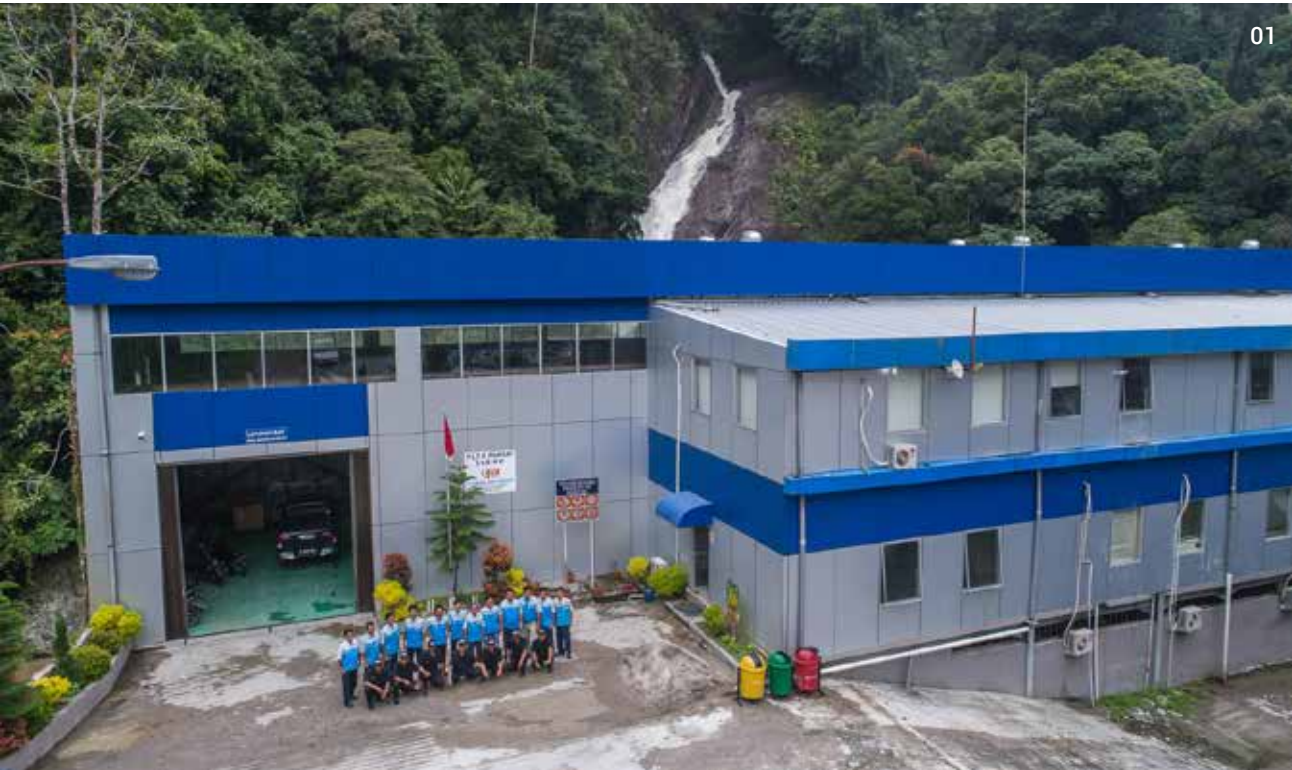
01. Exterior of Pakkat powerhouse 02. Turbine 03. Interior of cubicle room
