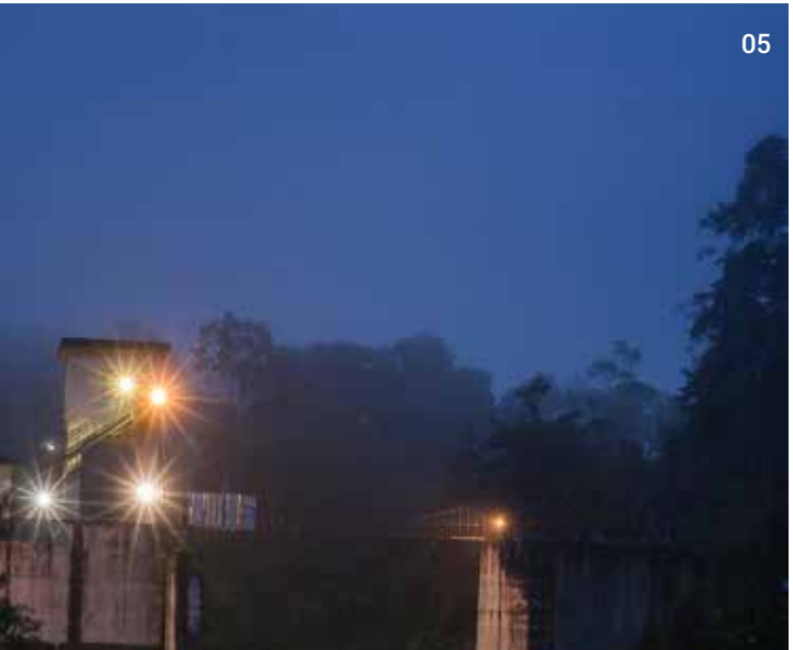
04. Turbine 05. Dam exterior
